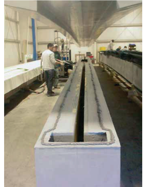
Technicians at Harbor Technologies dispense a bead of SCIGRIP SG230 HV adhesive on the composite bridge beam. The adhesive is used to structurally bond a composite top to the beam. The bulk metermix dispenser improved productivity by 50 percent.
